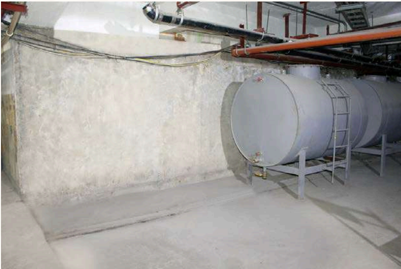
ON GOING SURFACE PREPARATION FOR WATERPROOFING WORKS
