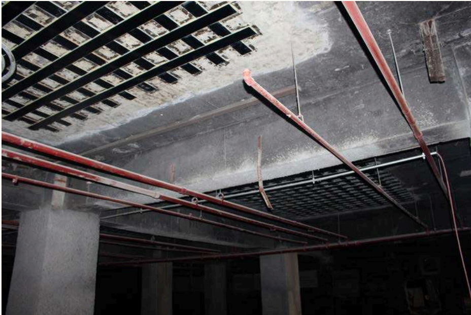
INSTALLATION OF CARBON PLATE
