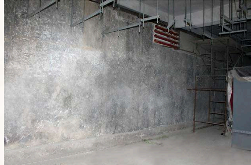
PLANTROOM SURFACE PREPARATION FOR WATERPROOFING WORKS
