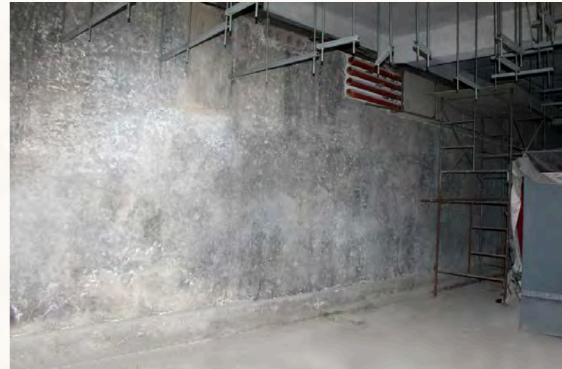
PLANTROOM SURFACE PREPARATION FOR WATERPROOFING WORKS
