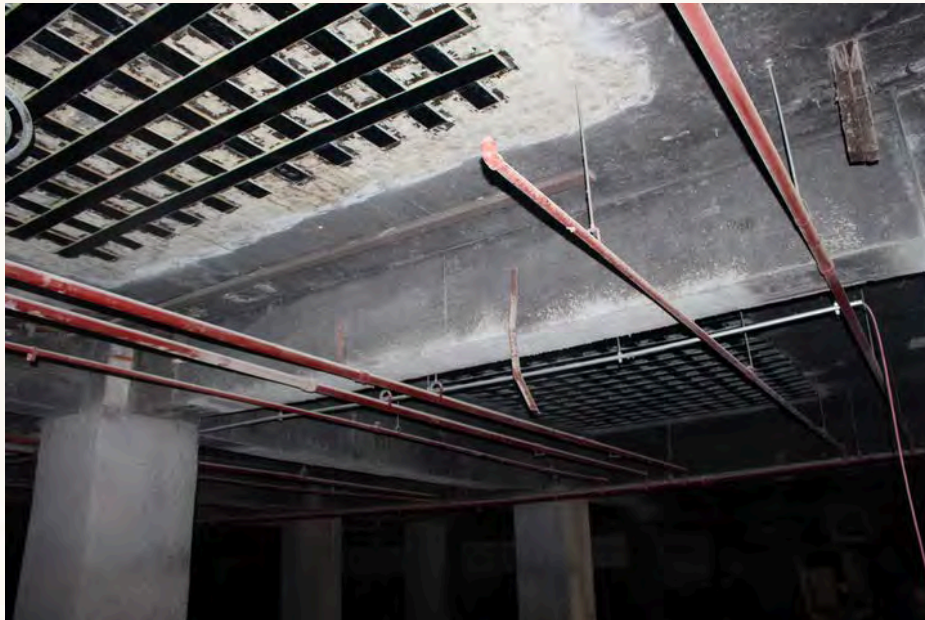
INSTALLATION OF CARBON PLATE
