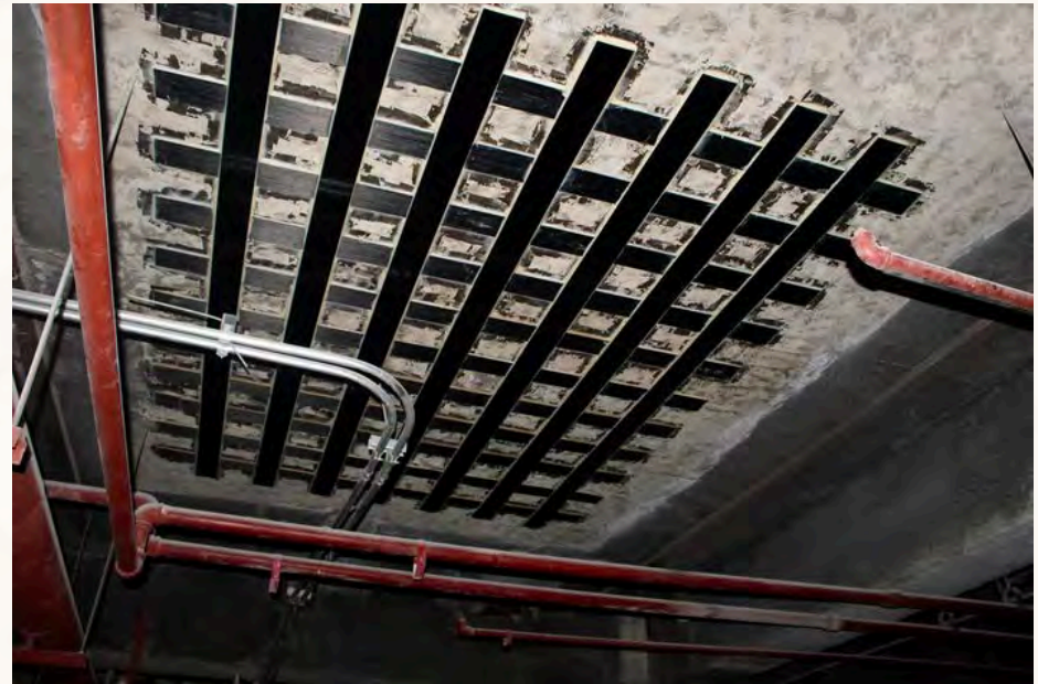
INSTALLATION OF CARBON PLATE
