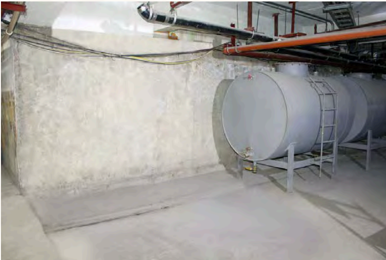
ON GOING SURFACE PREPARATION FOR WATERPROOFING WORKS
